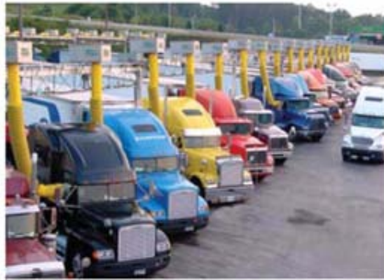
Trucks turn off their engines at a TSE facility and hook up to external air conditioning and power systems...
