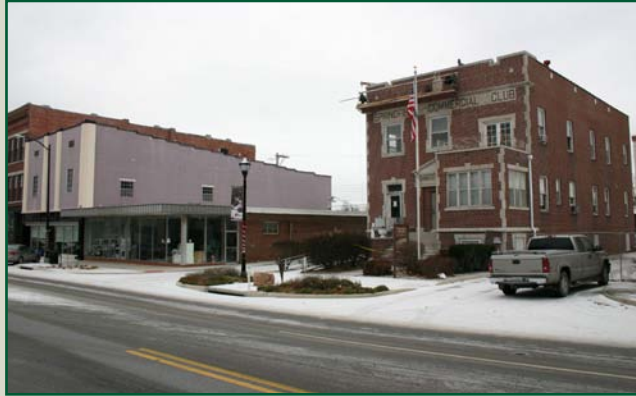
The historic Commercial Club Building in Springfield.
