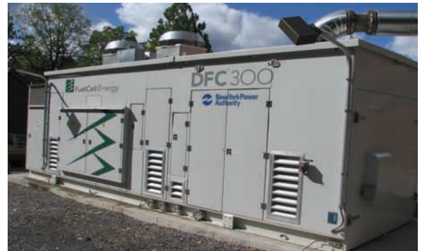
DFC 300A Molten Carbonate Fuel Cell
