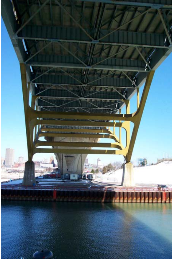
Milwaukee River passing under the I-794 bridge
