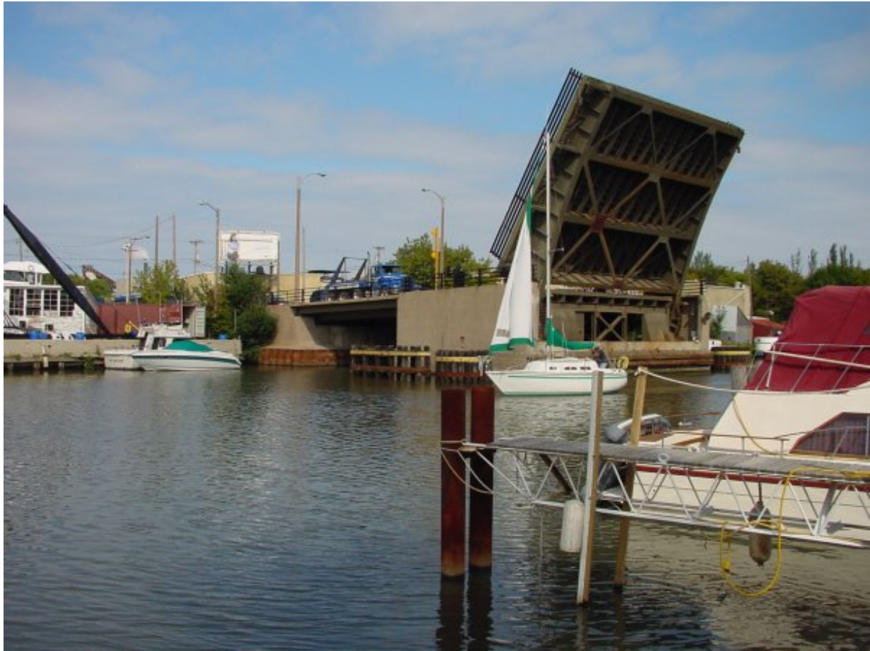
Bridge Lifts for Sailboat Passage on the Kinnickinnic River (photo courtesy of Wisconsin Department of Natural Resources)
