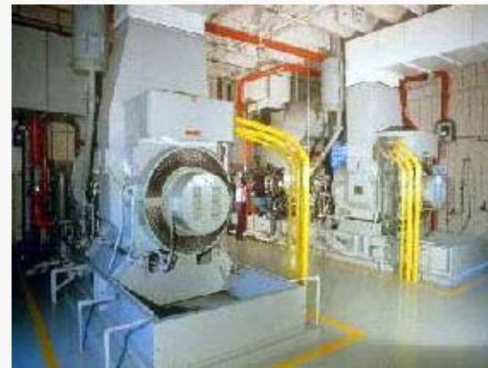
Gas Turbine (range from 800 kW to 10.5 MW)
