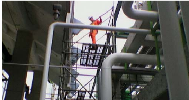
PEMEX engineer descends scaffold tower after taking wet seal measurements at a PEMEX gas processing center.
