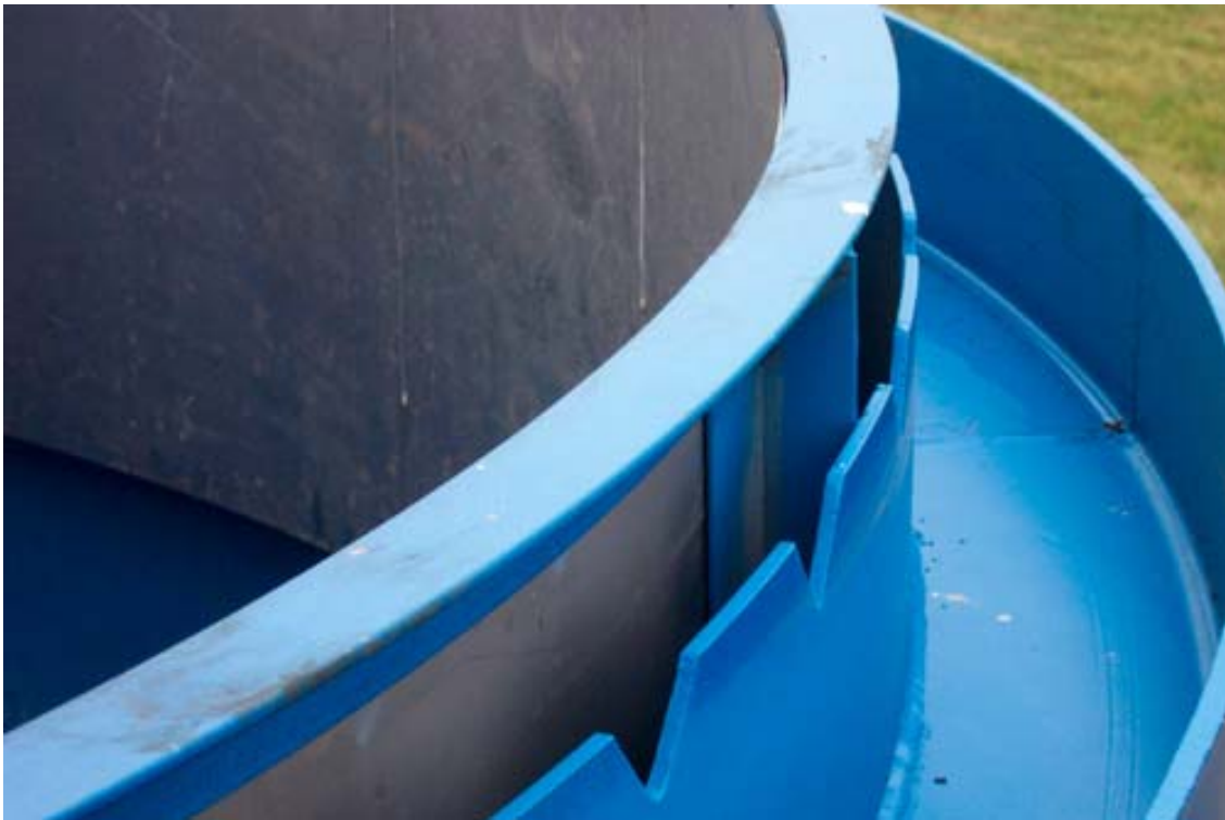
Figure 2-5. Effluent weir and baffle.
