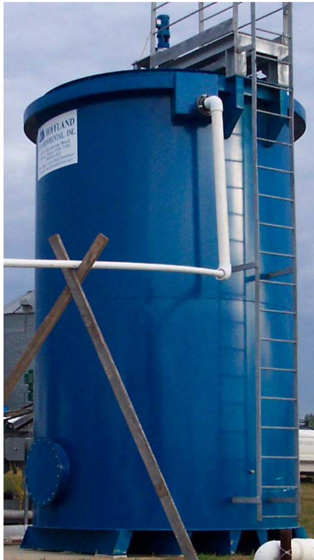
Figure 2-1. Hoffland Environmental Inc. clarifier.
