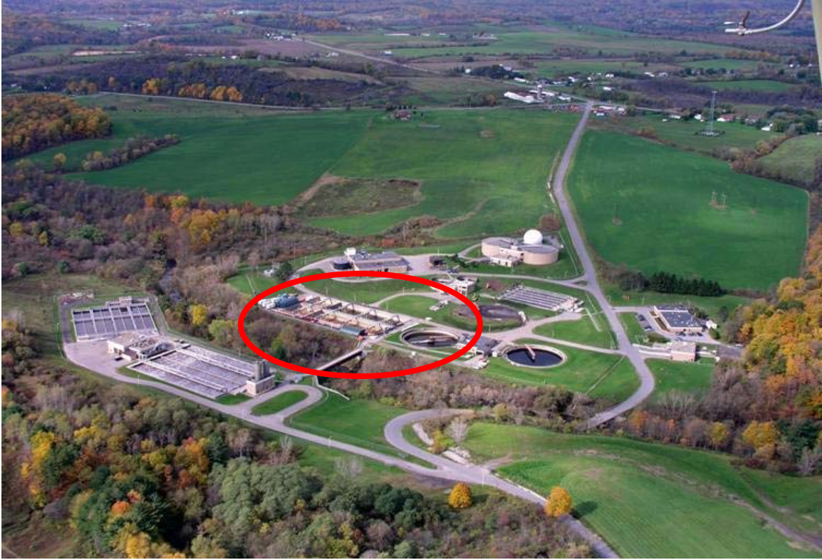
Figure 2-2. Aerial view of the Gloversville-Johnstown Joint Wastewater Treatment Facility and the UV Center.
