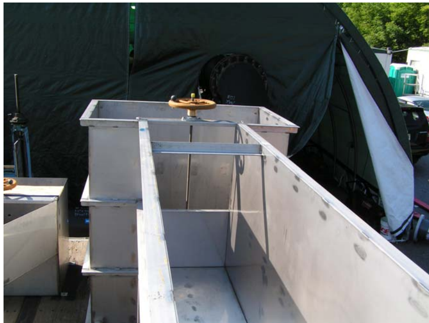
Figure 3-3. Influent stilling plate and effluent weir gate for the Siemens V-40R-A150 UV unit test channel.
