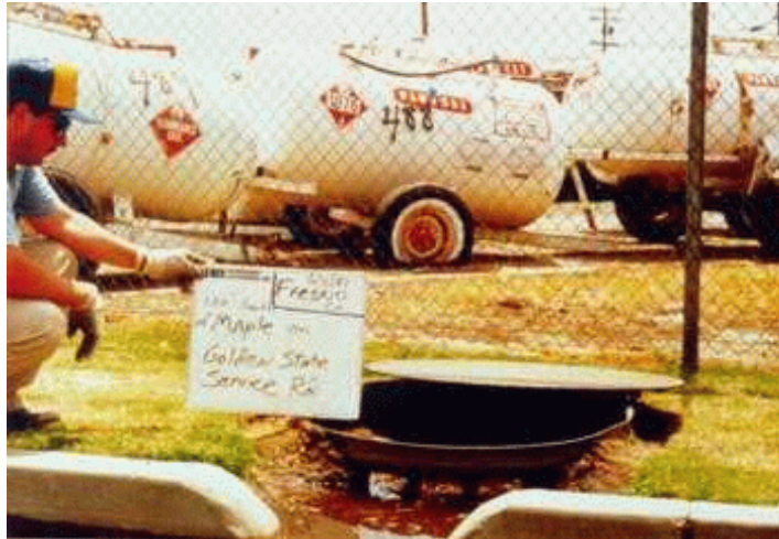
Figure 4. Storm Water Drainage Well in USEPA Region 5 (USEPA, 1999d)
