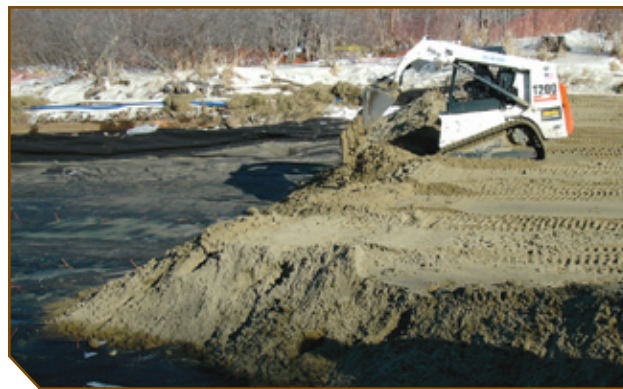
Figure 1: Installation of isolation cap at the Pine Street Canal Site.
