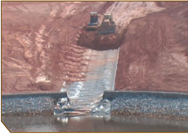
Barite Mine Site. Acid removal and waste-rock cap construction.
