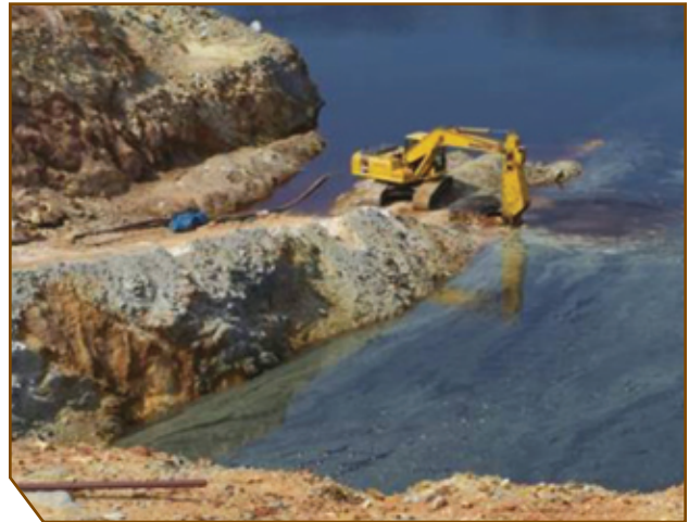
Barite Mine Site. Preparing the drainage area.
