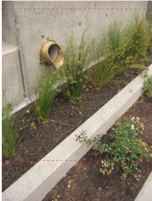
Figure 9. Disconnected downspout discharging to planter box.
