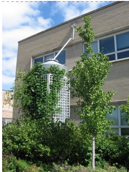
Figure 5. Rain water cistern.
