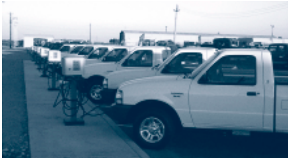
Figure 13 Cars charging at one of the sites of the current 29 charging stations installed around Vandenberg AFB. This particular site supports 12 charging stations along with 10 Ford Ranger EV truck applications for the 30th Civil Engineering Squadron.
