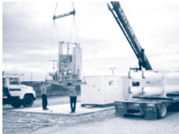
Figure 10 Construction of the CNG fueling station at Elmendorf AFB.
