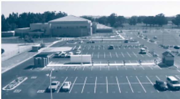
Figure 14 The parking island and charging stations that were constructed to accommodate Vandenberg AFB's SUVMS.
