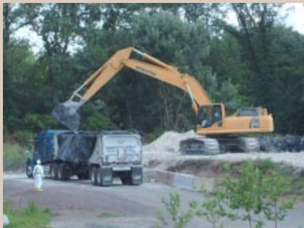
PVC sludge loaded for off-site disposal
