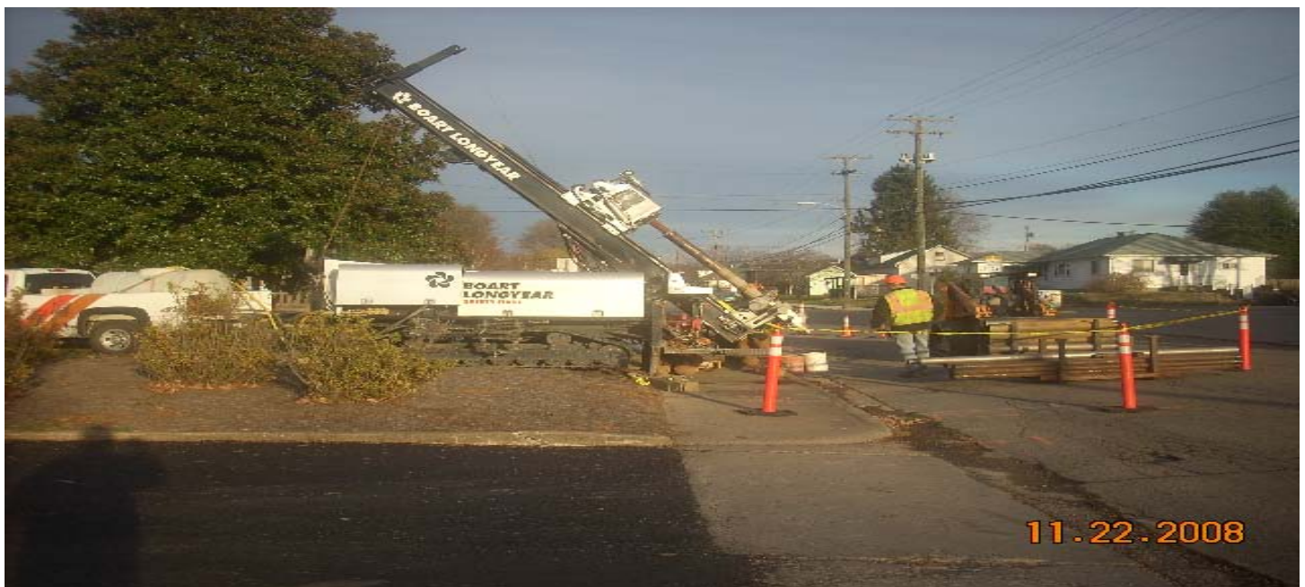
Typical well drilling operation
