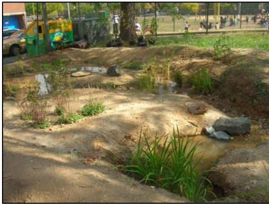
Photo 2. A constructed wetland at LaSalle Elementary.
