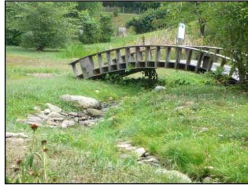
Photo 1. Lowell School daylighted a creek that runs through the schoolyard.
