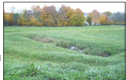
Constructed Wetland for treatment of milk house waste and manure runoff.
