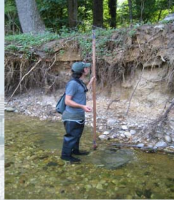
End results of excessive stormwater scouring: steep cliff erosion (undercut) is the result of too much stormwater coming too fast and scouring the stream banks in Oxon Run.
