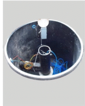
Manhole showing monitoring well MW-10D
