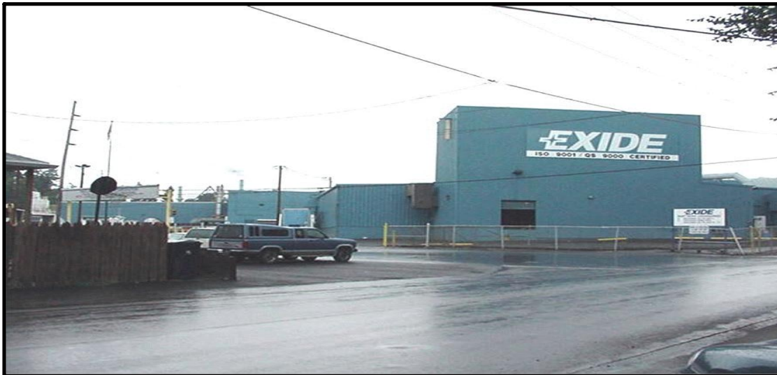
Figure 1 Exide Technologies, Laureldale, PA
