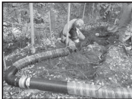
Excavation activities (November 2002, LEA).
