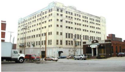
PCB Treatment Inc. 2100 Wyandotte – Kansas City, Missouri – Original Building
