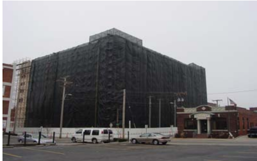
2100 Wyandotte – Kansas City, MO (Nov. 2004) Scrim with Scaffolding underneath for dismantlement
