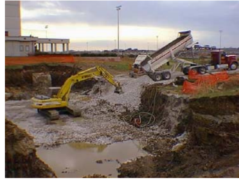
Excavating at Site ST 007, Former Underground Storage Tank Area
