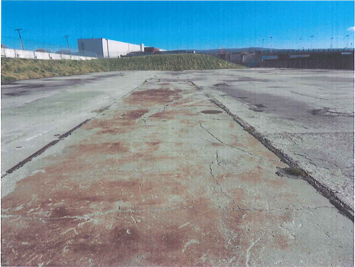
40s Slab Area – Looking East 11/9/11
