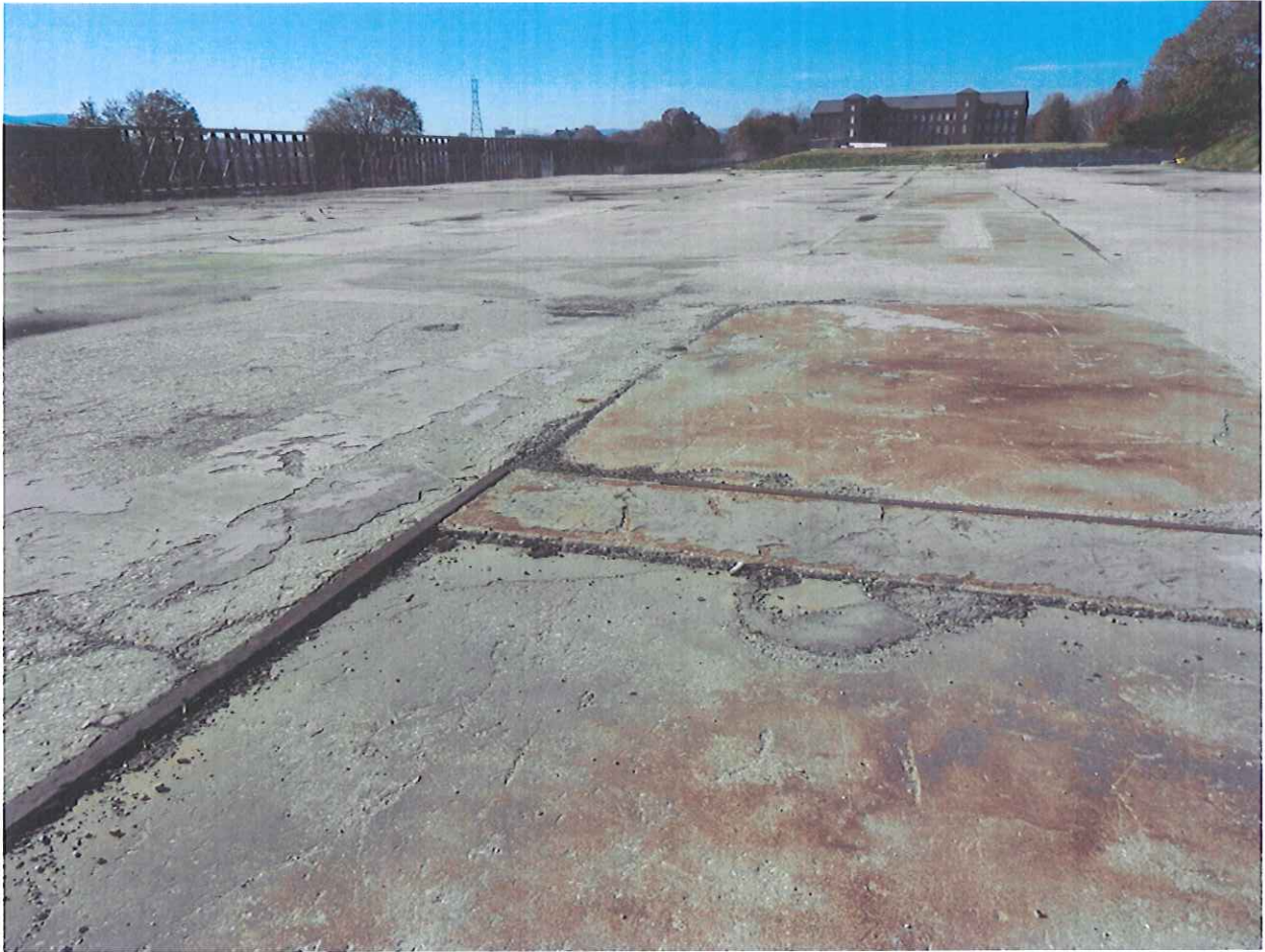
40s Slab Area – Looking West 11/9/11
