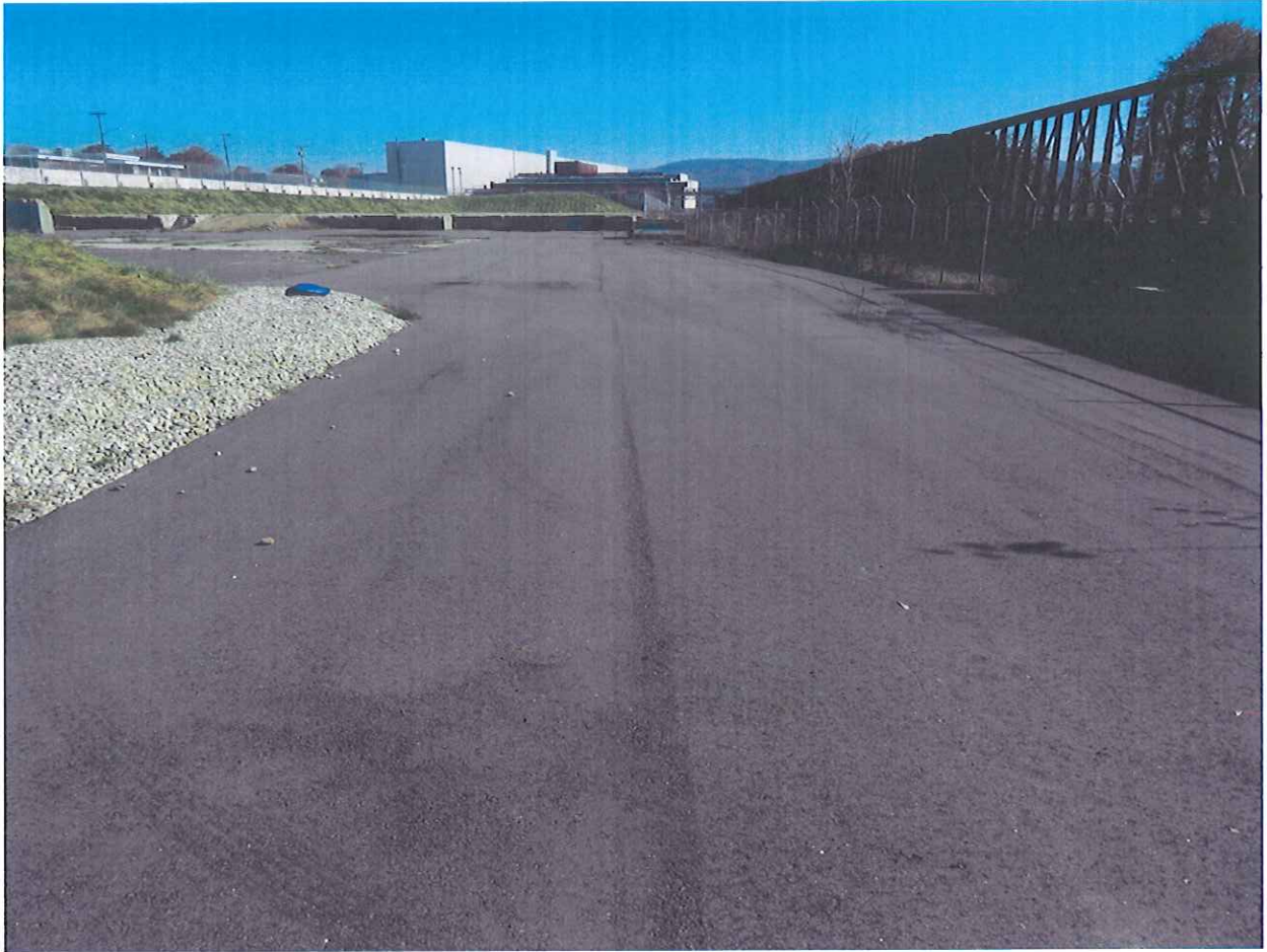
40s Other Ground Covering Feature Area 11/9/11
