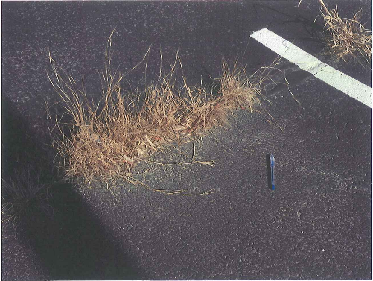
20s Building Demolition Barrier Area #1 Typical Vegetation Growth 11/9/11
