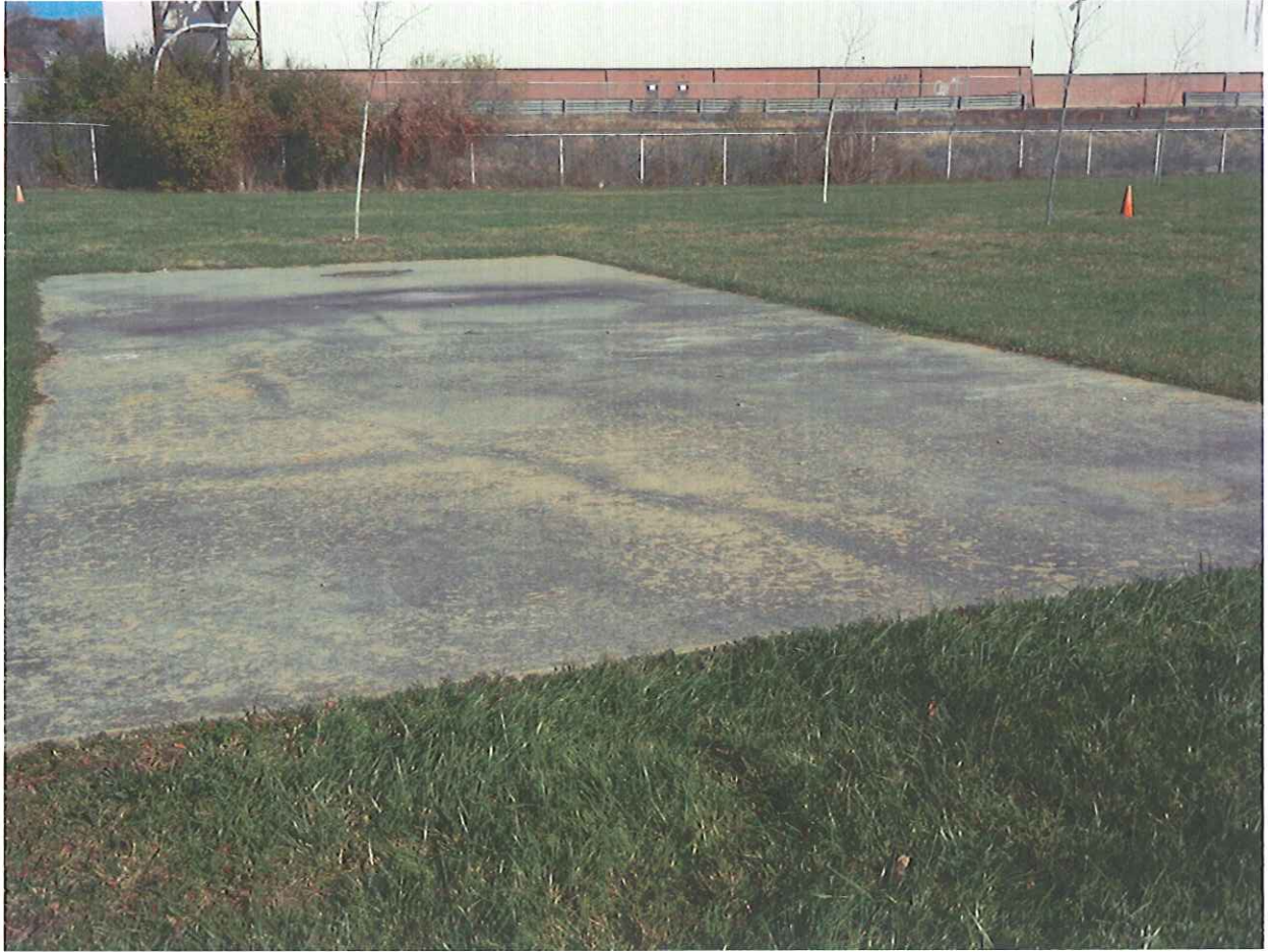
20s Building Demolition Barrier Area #2 View Looking North 11/9/11
