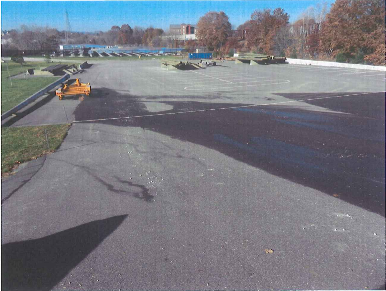
30s Building Demolition Barrier Area View Looking West 11/9/11
