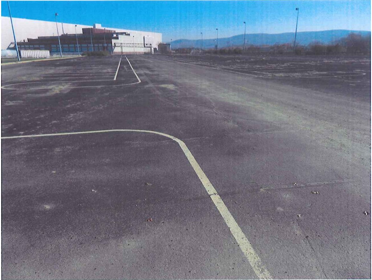
20s Building Demolition Barrier Area #1 View Looking East 11/9/11
