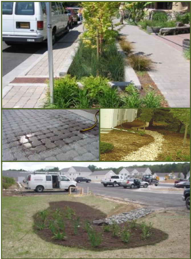
Figure 2. BMPs such as the bioretention, porous pavers, and infiltration trenches seen here are designed to provide water quality treatment and maximize runoff reduction through improved infiltration, evapotranspiration, and plant uptake. These are effective practices for reducing DCIA.
