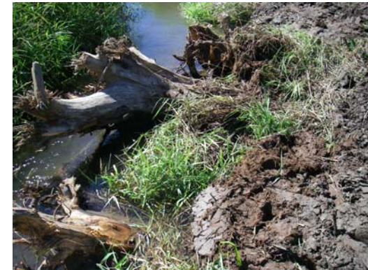
Large wood installation at the Mirror Lake Restoration Project
