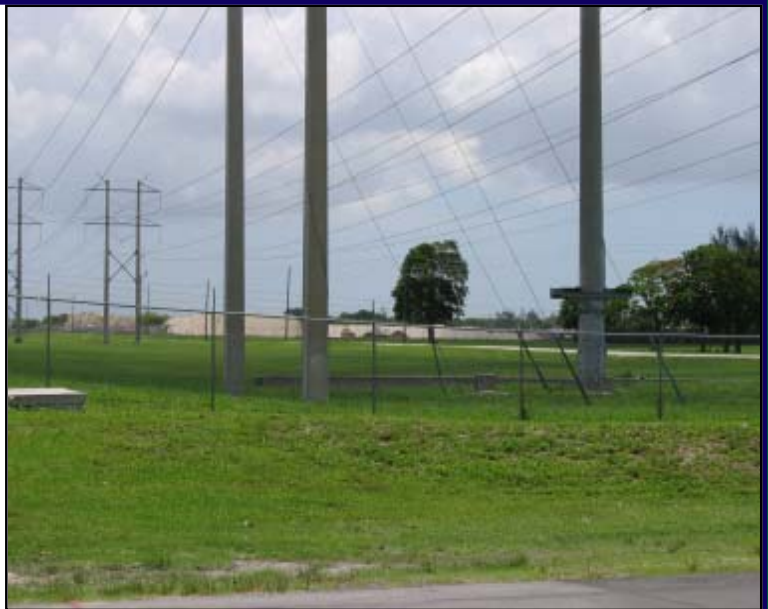
FP&L powerline easement with County buildings in background
