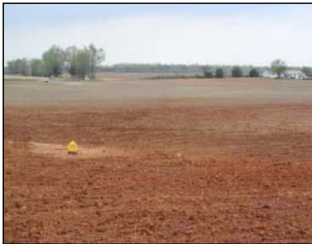
Newly installed sediment basin in the Brier Fork Watershed
