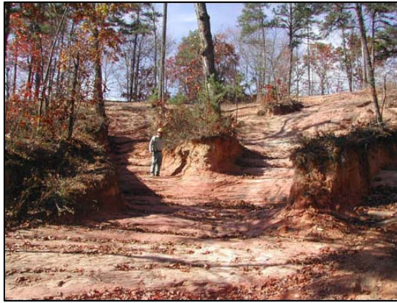
Ridge before restoration
