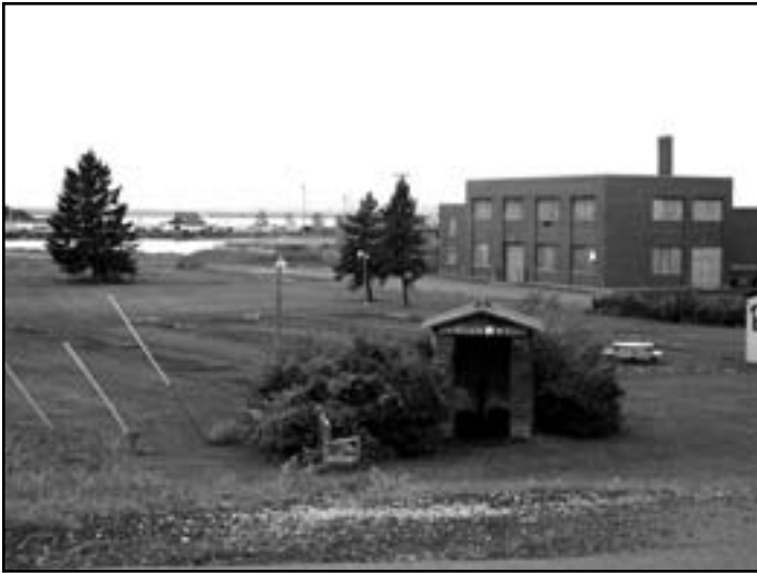
Closed artesian well and former wastewater treatment plant at Kreher Park.
