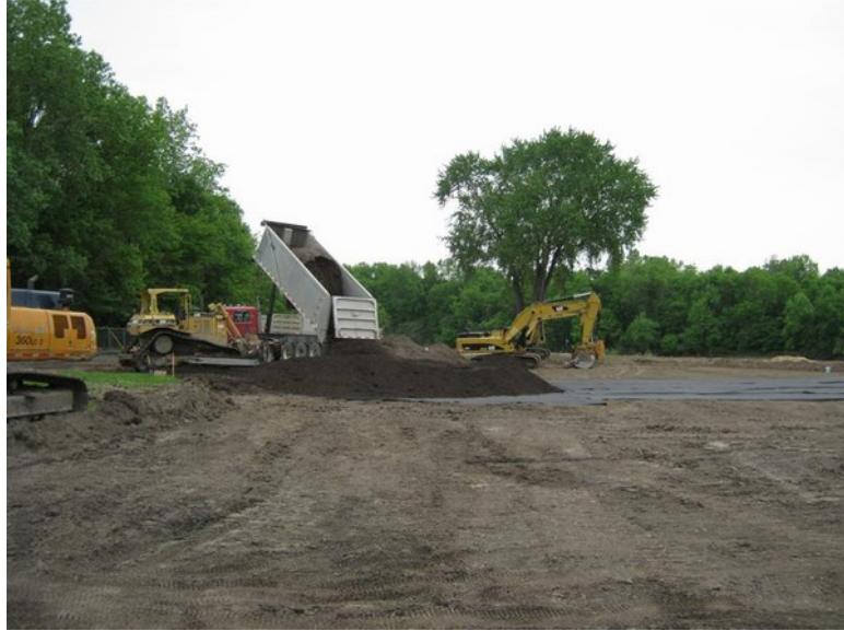
Backfilling activities, May 26
