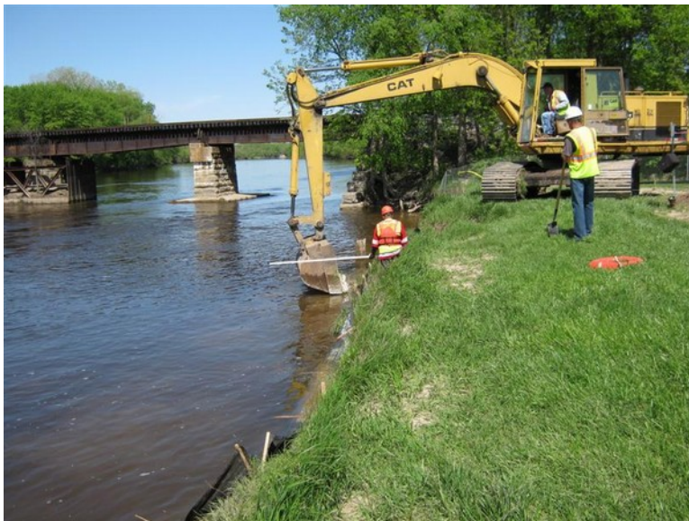
Placing silt curtains in the river, May 18
