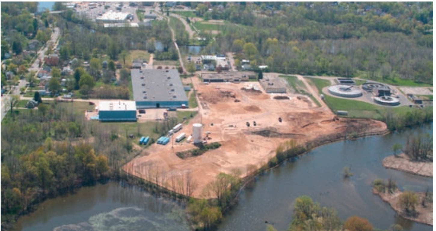
Photo 2: View of the Site facing South (May 2006).
