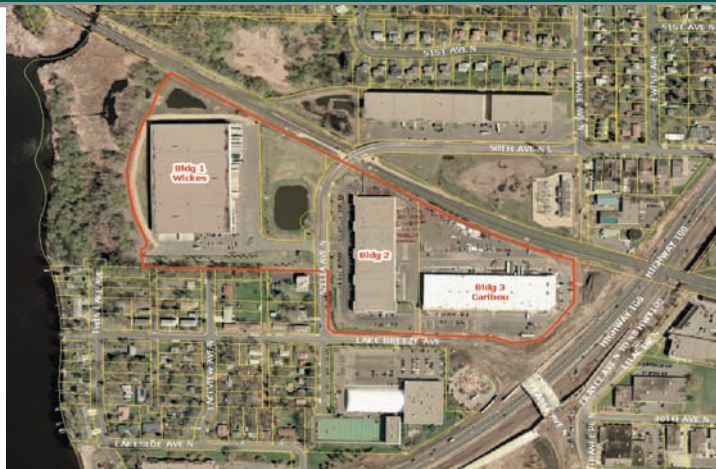
An aerial view of France Avenue Business Park
