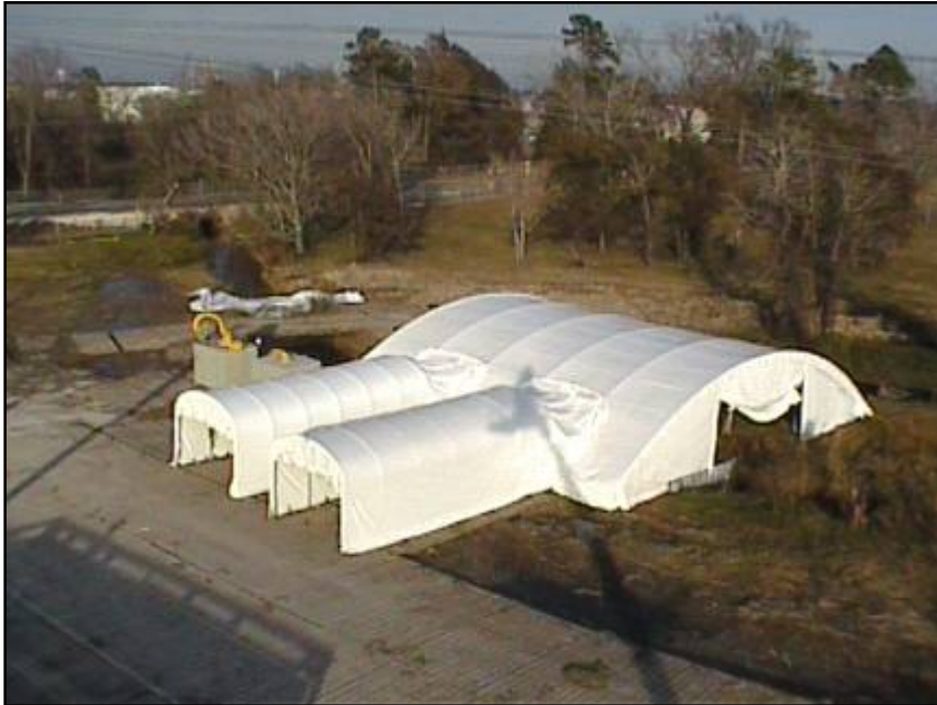
Containment Structure over West Ditch
