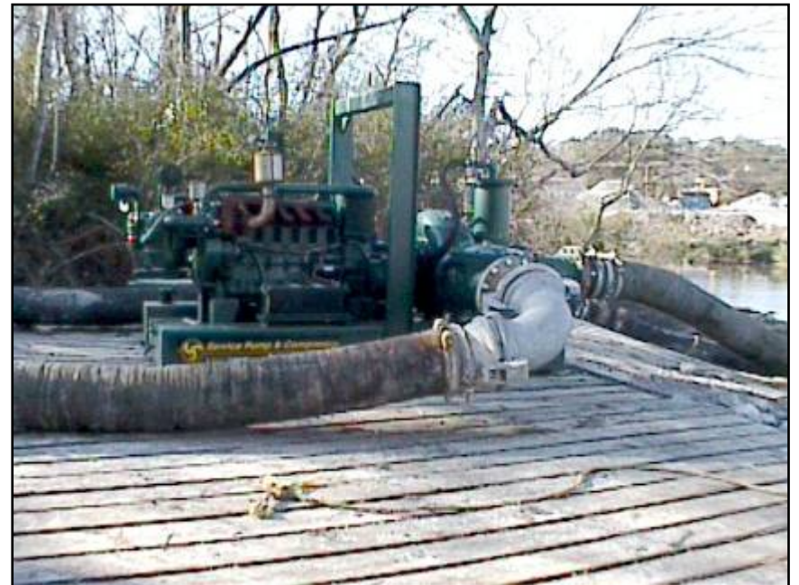
Pumps Re-routing Bayou Verdine
