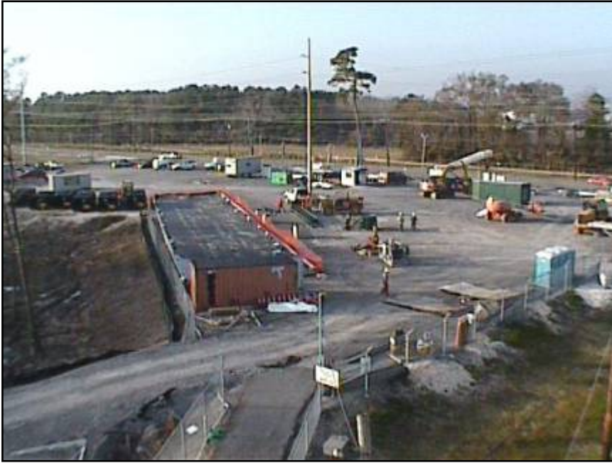
Project Work Area
