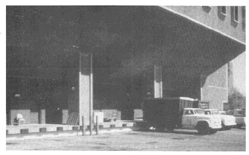
Exhaust fumes are drawn into this building's outdoor air intake when trucks are idling at the nearby loading dock. Tools such as the Occupant Diary and Log of Activities and System Operation can help to identify intermittent pollutant sources such as this one.
