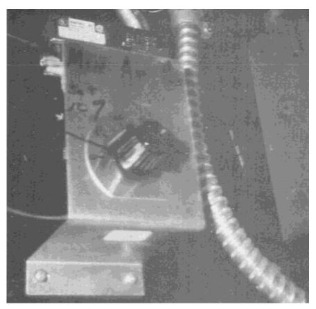
The design specifications for this building called for a minimum 20% setting on the outdoor air damper control. Facility staff lowered the minimum outdoor air setting to 10% in order to save energy and reduce operating costs. As a result, the building was underventilated whenever outdoor temperatures were either very hot or very cold.
