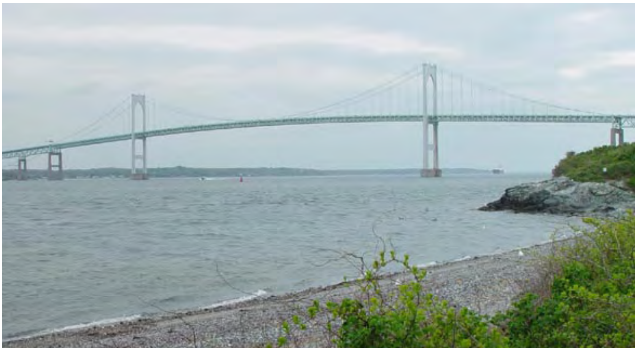
Newport Bridge, RI (courtesy of NBEP).
