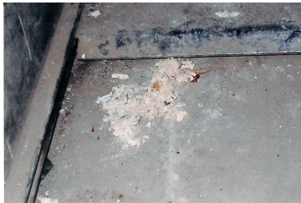
Regulated asbestos containing material pipe insulation debris.
