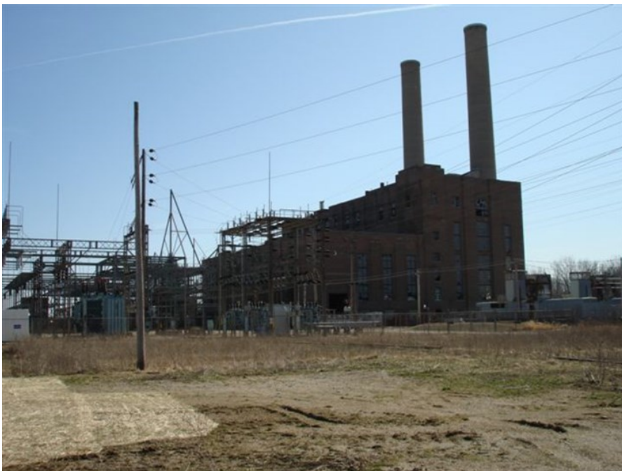
The Morrow Power Plant was the former power generation facility in which asbestos material was illegally stripped and removed
