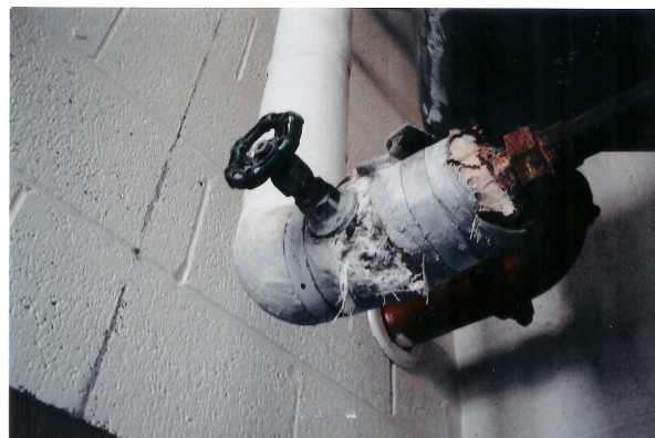
Regulated asbestos containing material wrapped steam pipe attached to a heater suspended from the ceiling.
