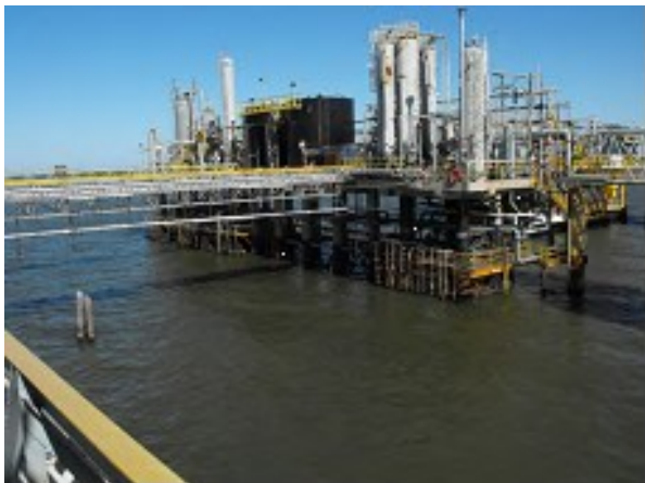
Well site platform and flow lines
