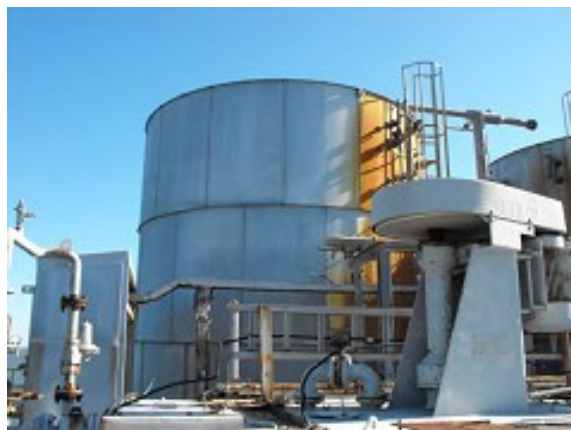
Offshore storage tanks
