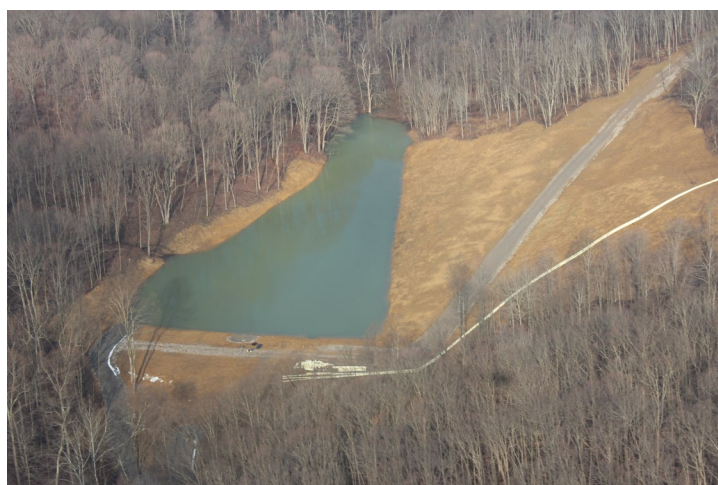
The impoundment for the Goshorn well pad constructed in 2011. The white pipe at the bottom leads from the impoundment to the well pad.
