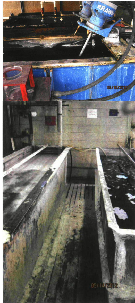
Inspection photos from inside Southern California Plating Company.
