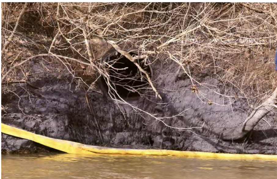
The coal ash discharged into the Dan River from this broken 48-inch storm water pipe.
