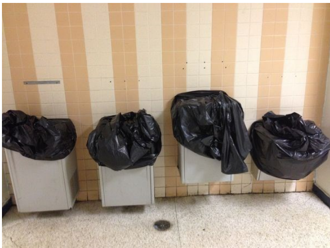
Drinking water fountains covered up as a result of the defendants falsifying water testing logs.
