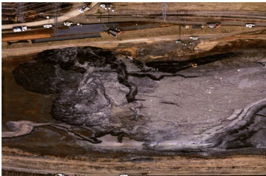
The primary coal ash basin at the Dan River Steam Station with all the wastewater drained out as a result of the pipe collapse.
