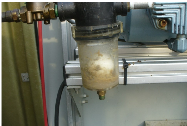
An interceptor effluent line clogged with the illegally disposed waste grease.
