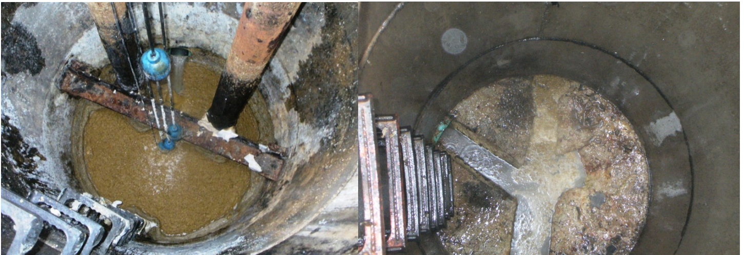
Pumping stations clogged with the illegally disposed waste grease causing significant damage to the pump stations.
