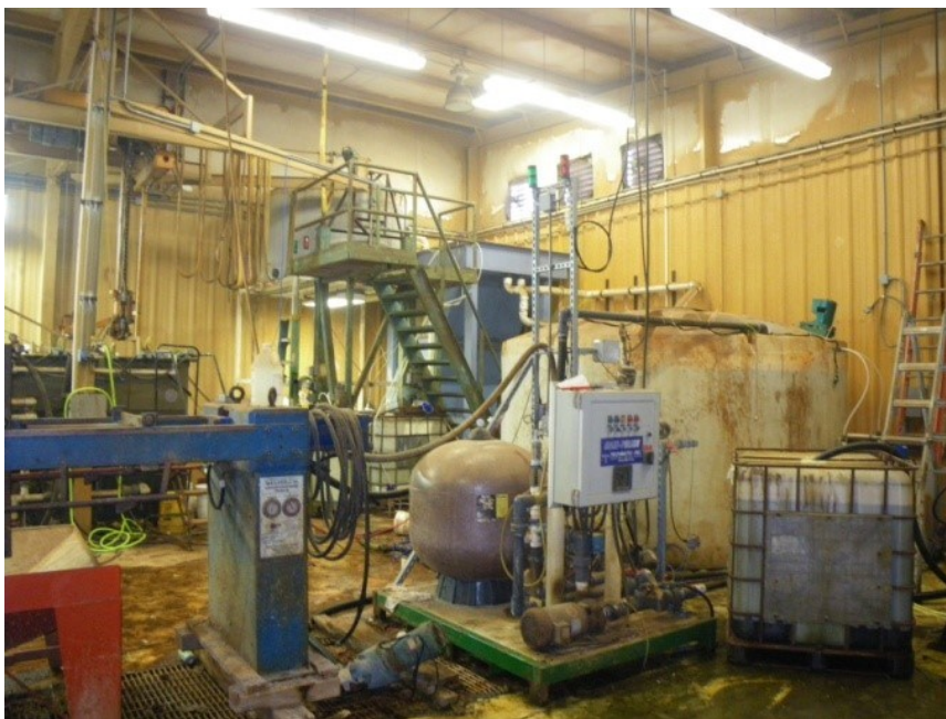
The treatment system inside C&R Plating
