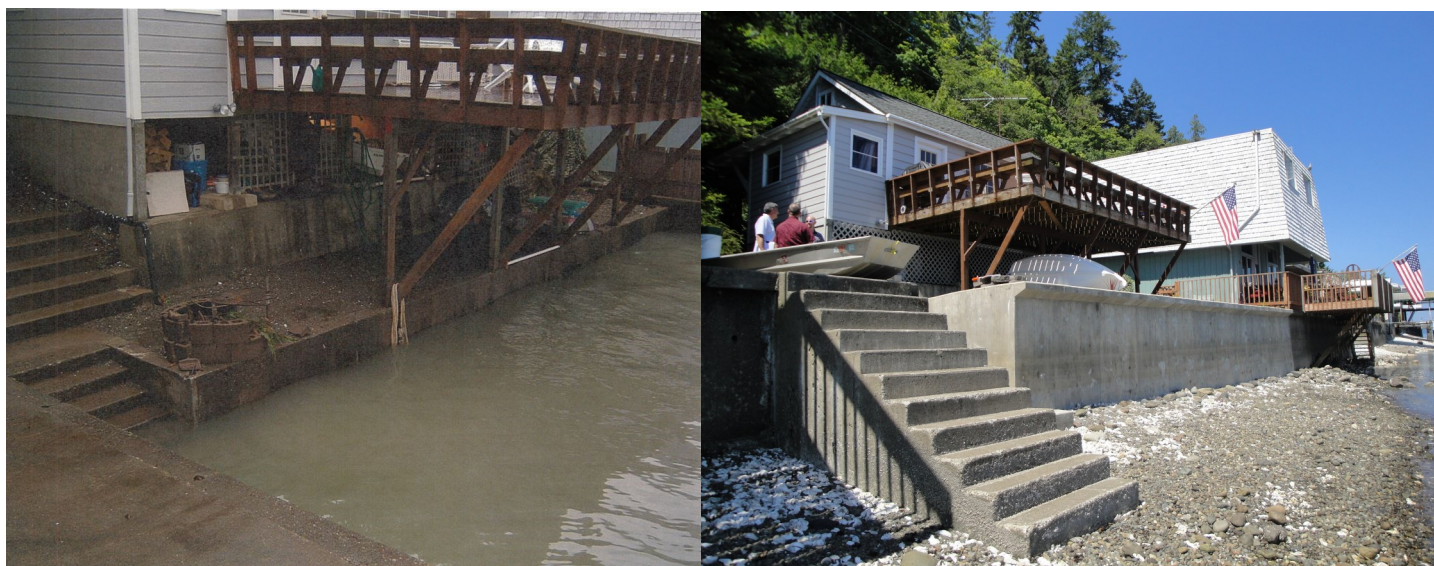
More photographs of Koloski's beachfront property before construction of the bulkhead (left) and after (right).
