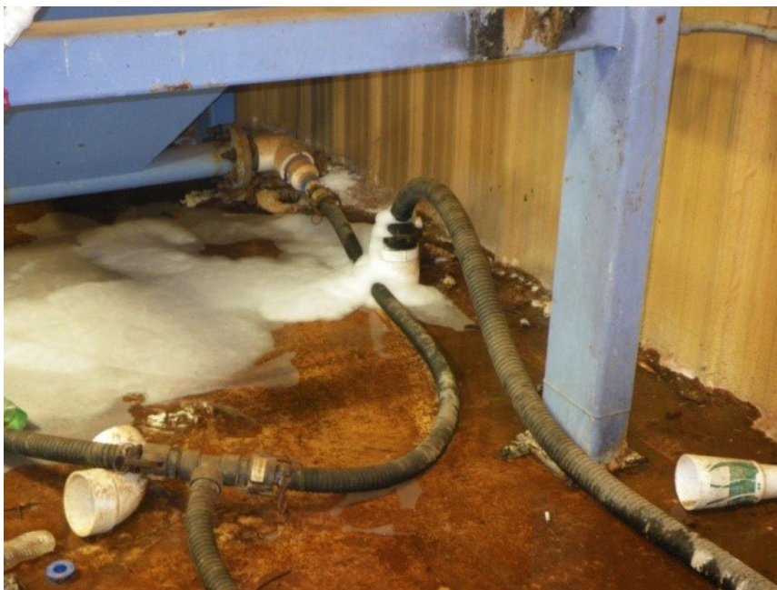
Hoses in C&R Plating leading to the drain and city sewer system.
