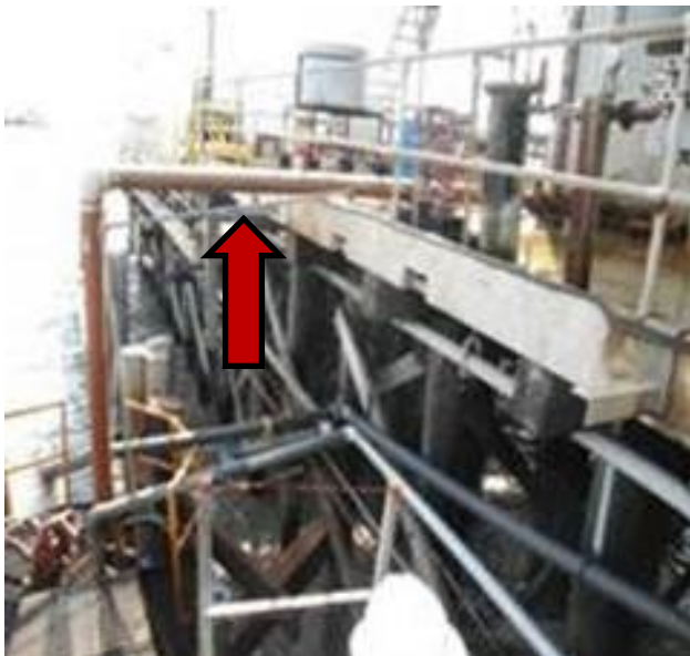
Discharge pipe (shown with 90 degree angle).
