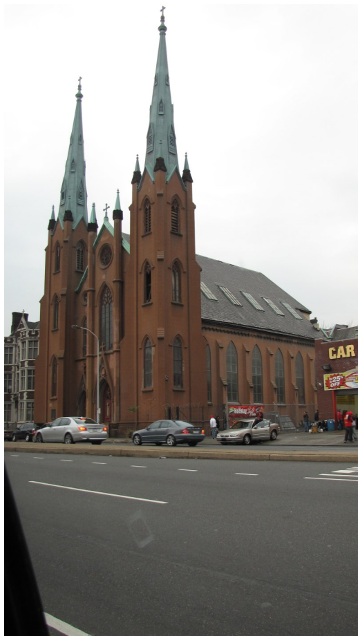
Former church where illegal asbestos removal was conducted.
