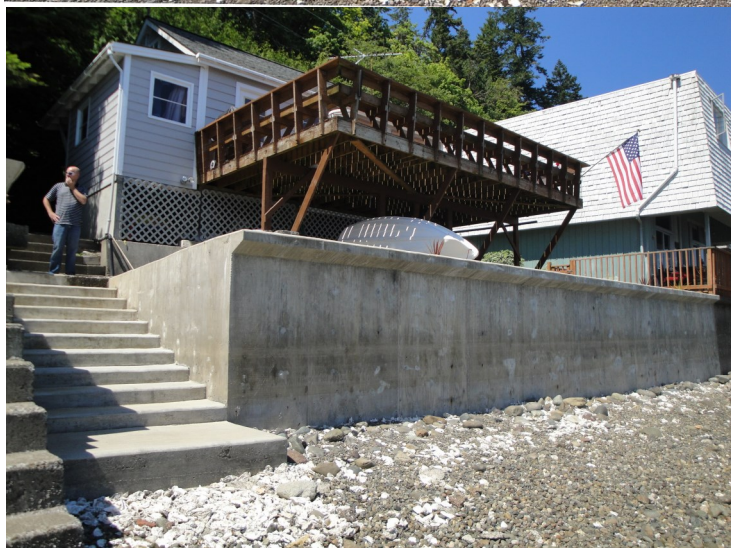
Koloski's beachfront property before construction of the bulkhead (top) and after (bottom).
