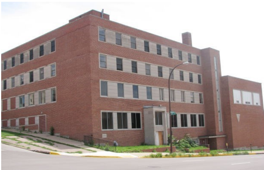
The old YMCA building from which Wolf, and others at his direction, tore and removed pipes containing asbestos.
