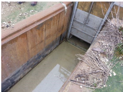
Picture of the open gate on a storm water culvert leading to Bayou Casotte.
