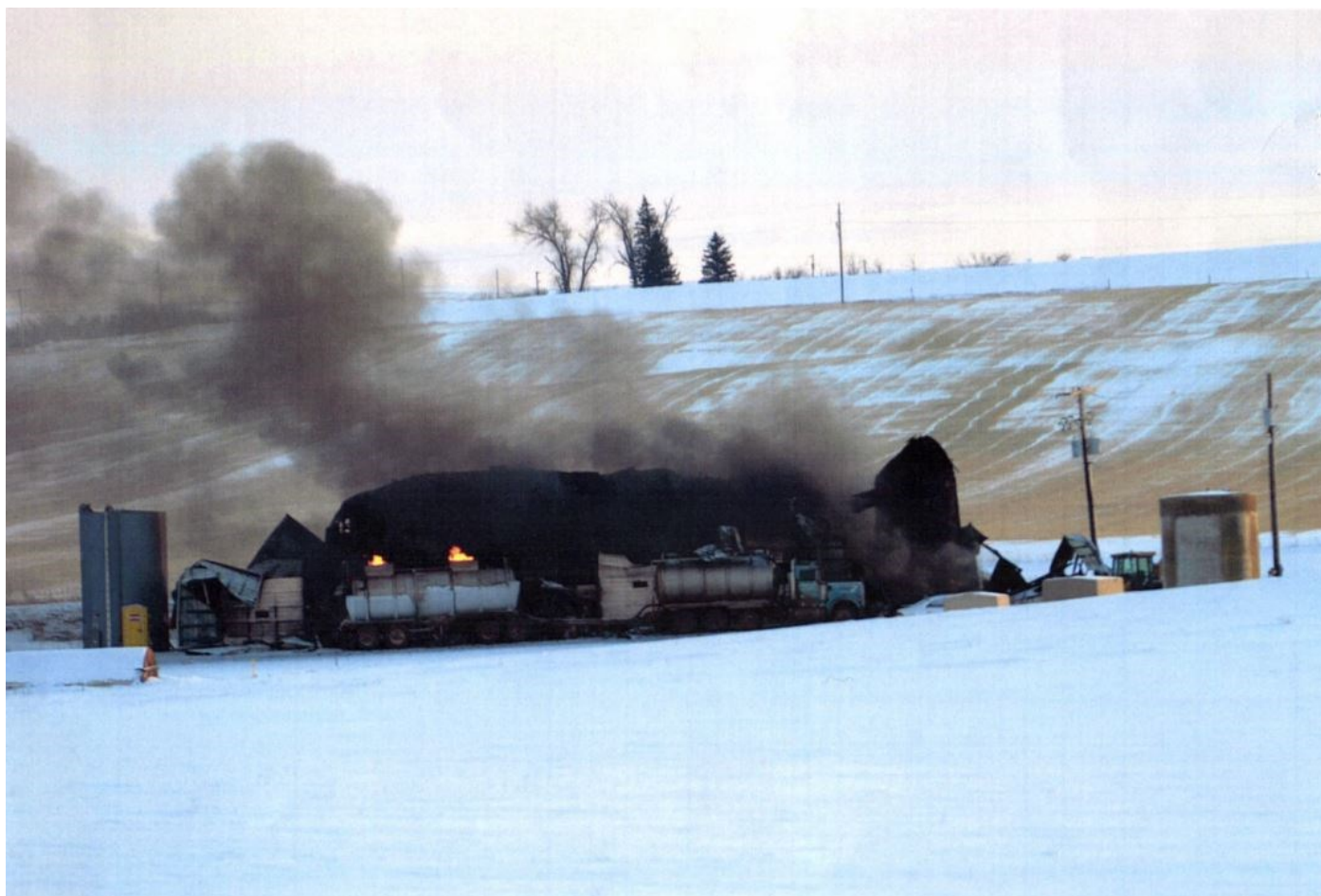
The fire that ignited while Steen was pumping from the truck he drove into the Custom Carbon Processing facility.
