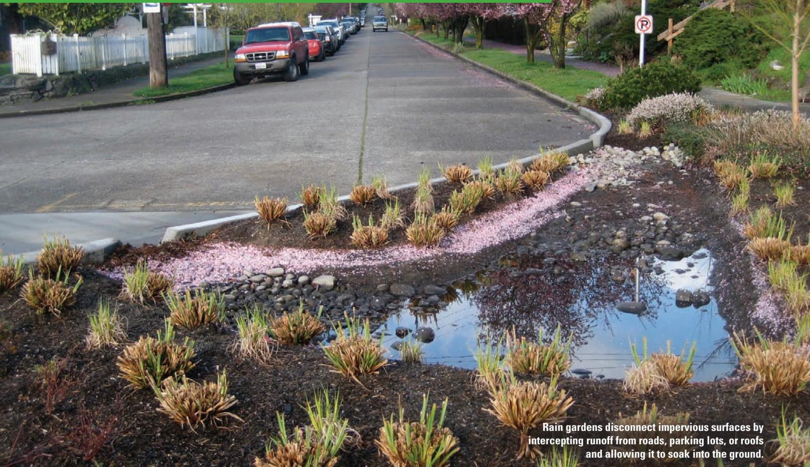
Rain gardens disconnect impervious surfaces by intercepting runoff from roads, parking lots, or roofs and allowing it to soak into the ground.
