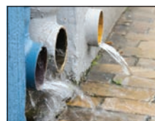
EPA green infrastructure researchers provide key tools, such as the National Stormwater Calculator, to address stormwater management.
