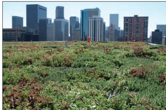
Green roofs can be used effectively to reduce stormwater runoff from commercial, industrial, and residential buildings.
