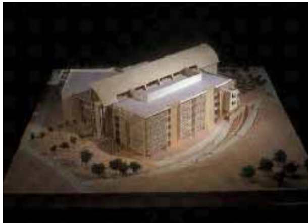
Figure 4.2 CSUMB Library - Concrete Frame
