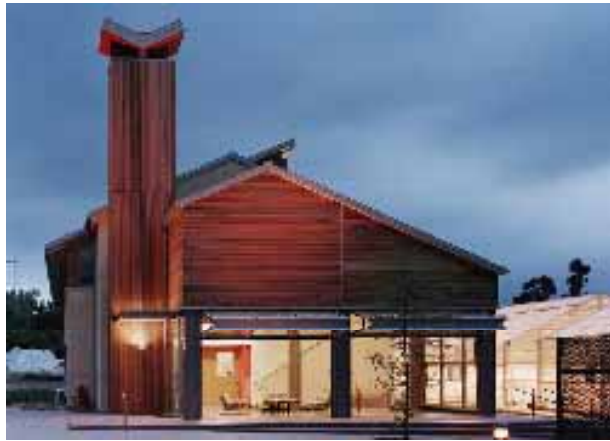
Figure 4.1 Global Ecology Research Center - Steel Frame
