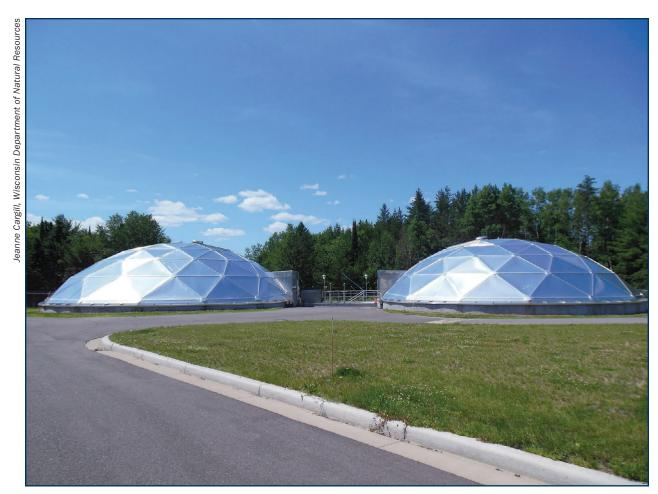
Aluminum dome covers on the two primary clarifiers at the new wastewater treatment plant (WWTP) in Rhinelander, Wisconsin.
