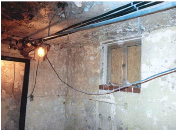
Asbestos-containing pipes in building
