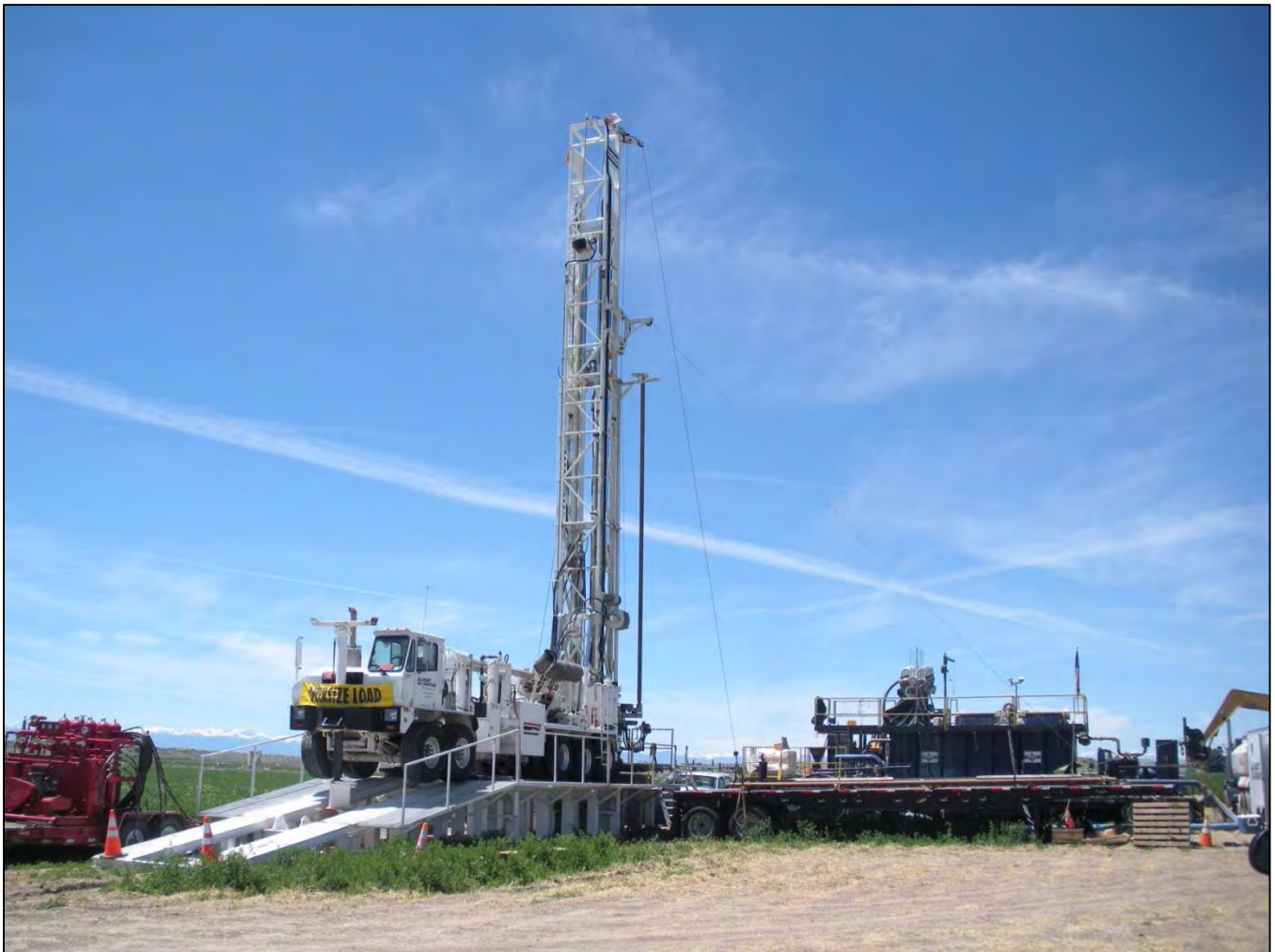
Figure C1. Photograph of drilling rig on platform with shakers for mud recirculation at MW02.
